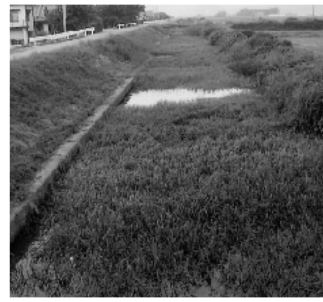
承水溝の現状
